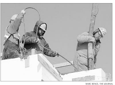
Workers with SBC Construction use a cement boom to fill the walls of a newly constructed home in Leduc.
