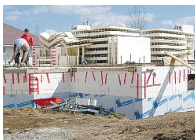
Super-solid construction of Dabro’s Wetaskiwin showhome includes poured concrete and rebar.
